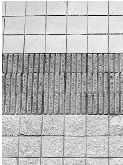
Figure 2-9 Smooth, split-ribbed, and split-faced concrete block.
